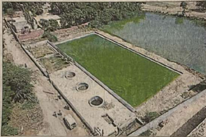
The Thapar model of three-well wastewater management system at Bhai Bakhtaur village in Bathinda district.
